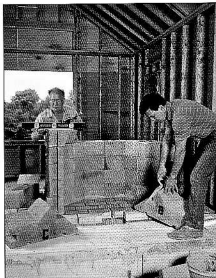
The molded masonry components form the firechamber of the Radiant Fireplace. This modular design insures proper fireplace construction, consistent quality and optimum performance.
