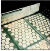
The honeycomb-shaped ceramic grate increases the efficiency of the boiler, since it was developed to bring in the primary combustion air and is provided with air inlet openings. Through substitution of insert stones with air inlet openings by stones without openings, the quantity and pattern of incoming air under the glowbed can be regulated and the boiler can be adjusted to various shapes and types of wood fuel.
