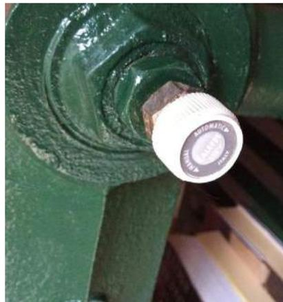
Hygroscopic air vents contain a special cellulose fiber disc that, when dry, allows air to pass through it and exit the vent. When moisture reaches the disc, it expands very quickly to stop further flow from the device. The location and thickness of the fiber disc is illustrated in Figure 2-18.
