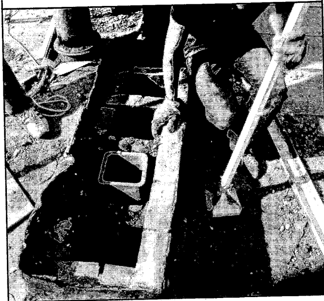
Above: This section of clay liner has been buttered with refractory mortar. It will be lowered onto another, similarly coated section, and will have another section lowered onto it. Below: In this photo, you can see that the chimney stack has four flues, only one of which is being lined.
