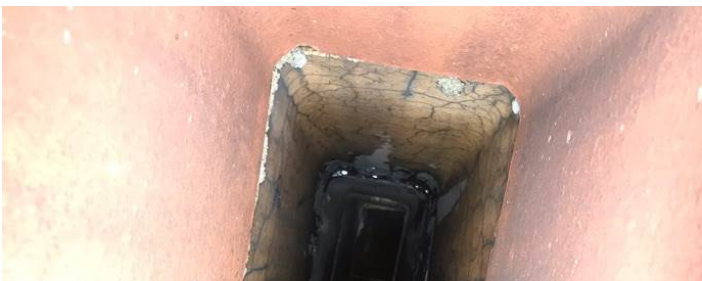
Notes: Remove old calk and remortar (pitch out)
