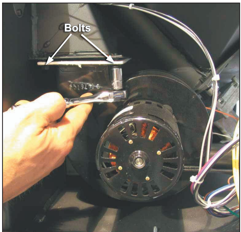
Figure 27: Removing The Convection Blower.
