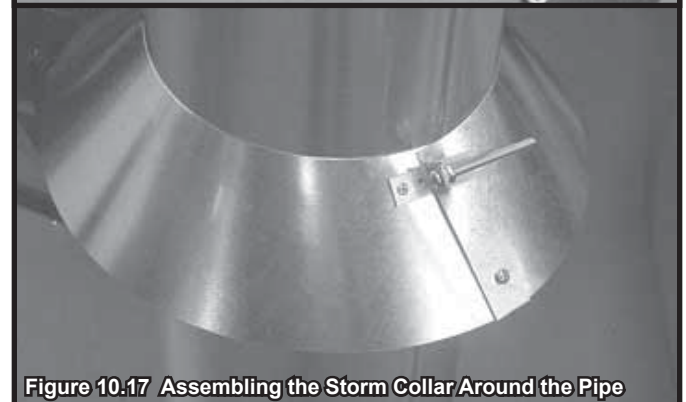
Figure 10.16 Assembling the Storm Collar
