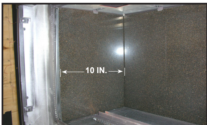
Figure 13. View of Back and Side Pieces Installed.
