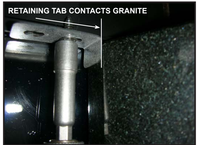
Figure 21. Placing Outer Corner Granite Trim Piece.
