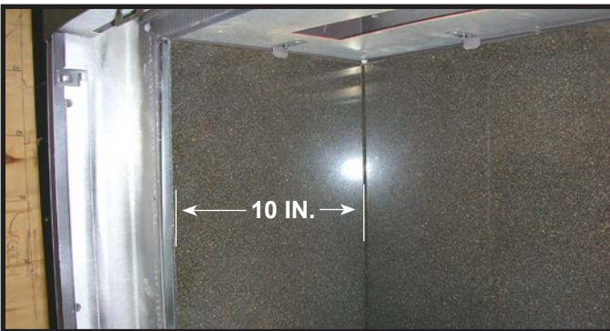
Figure 8. View of Back and Side Piece Installed.
