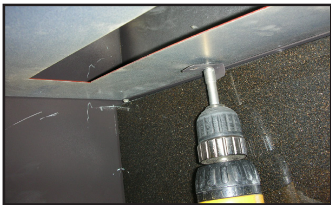
Figure 12. Fastening Angle Tabs to Secure Granite in Place.
