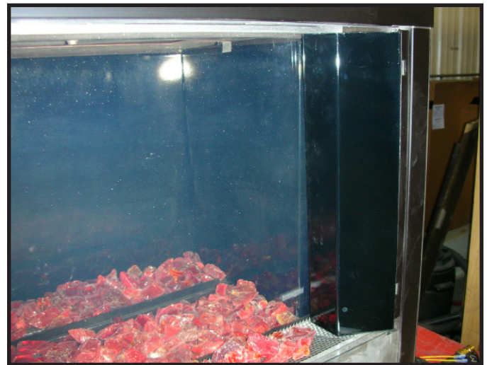
Figure 11. Installing Outside Corner Trim Piece onto Clip.
