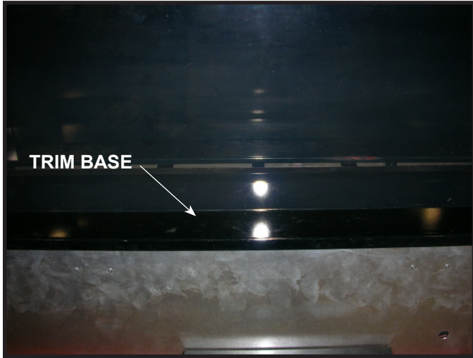
Figure 14. Porcelain Trim Base Installed.
