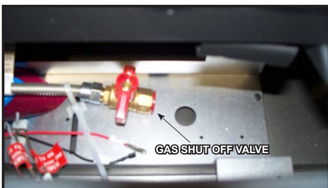
Figure 11.4 Gas Fitting Access
