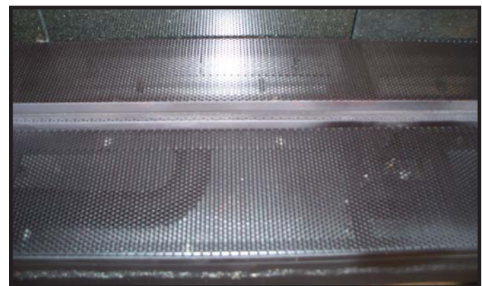
Figure 15. Base Mesh Installed.
