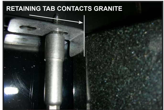
Figure 10. Placing Outer Corner Granite Trim Piece.
