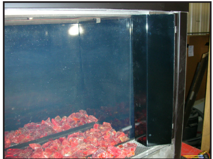
Figure 10. Outside Corner Trim Piece Installed.
