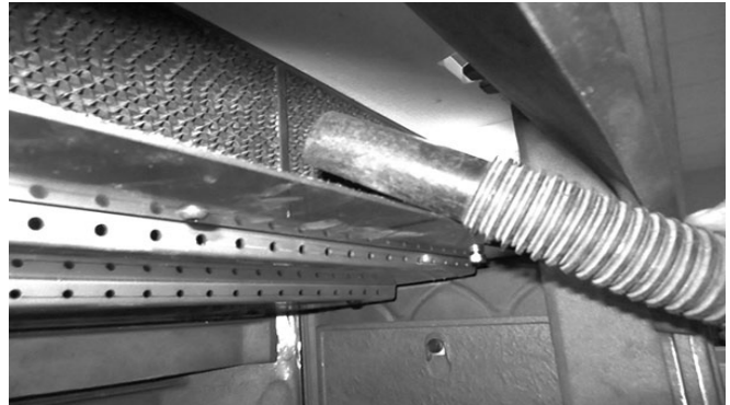
Fig. 18. Vacuum the combustor cells after brushing.
