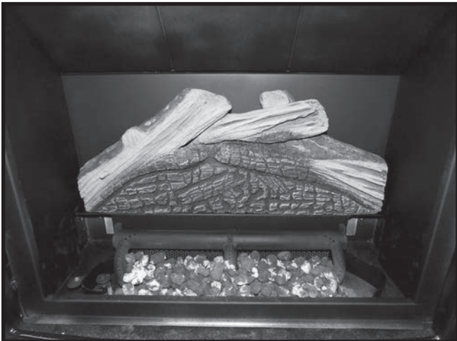
Fig. 42 First log set in place
