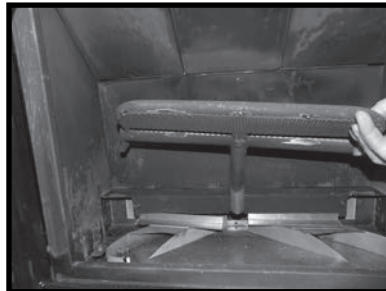
Fig. 68: Burner insertion onto the orifice
