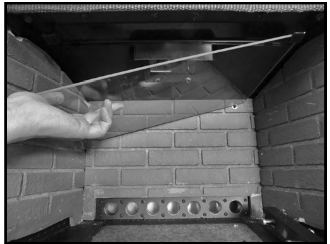
Figure 31: Inserting baffle into the upper corner.
