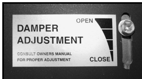
Figure 46: Damper adjustment indicator.
