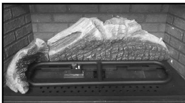
Figure 76: Rear Log Installation
