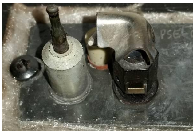
Figure 30 – Pilot in LP (slide gate to rear of Pilot Tower)
