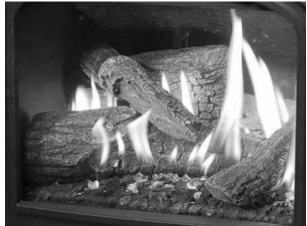
Figure 41 – Typical Burner Flame Appearance
